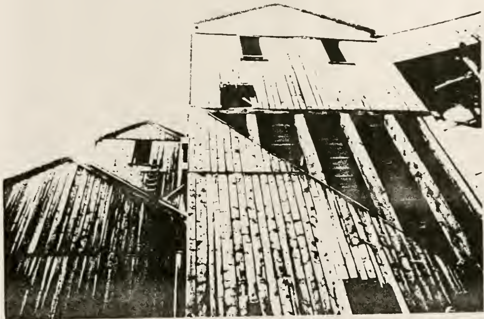
Figure 84. Revenue Mill (structure #34), north view.
